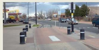
Pedestrian access to transit is supported in many parts of Boulder through surface treatments like raised crossings and wider sidewalks.
