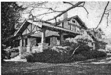
Style Craftsman Address 721 Spruce Street Architect 1913 Date Unknown Name Armstrong House
