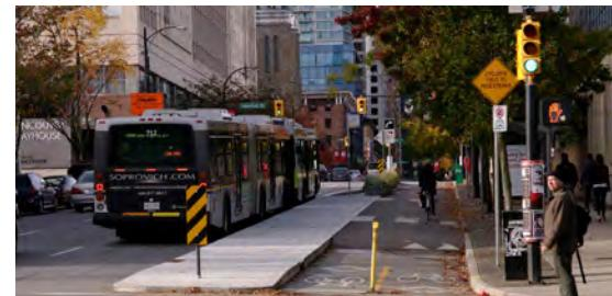
The Dunsmuir Separated Bike Lane in Vancouver BC is an example of a separated cycle track with a sidewalk that is clearly defined from the cycle track, and a bus stop with defined transitions to the sidewalk for safe pedestrian movement.
