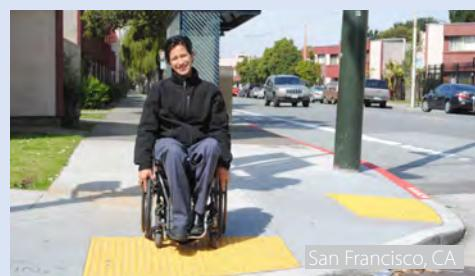
◀ **Universal Design:** Intersections should provide facilities that can safely move people of all ages and capabilities across the street. Design elements like curb ramps, level landings and gutter seams, visible and audible signals, smooth surfaces, accessible push buttons (or default WALK phases), and signage that may help pedestrians navigate intersections should be integrated into intersection design.
