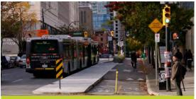
The Dunsmuir Separated Bike Lane in Vancouver BC is an example of a separated cycle track with a sidewalk that is clearly defined from the cycle track, and a bus stop with defined transitions to the sidewalk for safe pedestrian movement. mage from Flickr user pwkrueger
