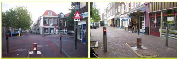
Electronically-activated bollards allow buses or deliveries access to the Delft, NL city center, which is otherwise a pedestrian and bicycle-only zone. Image from nl2011transpo
