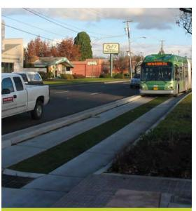
A raised concrete barrier provides physical separation between the roadway and the curbside bus lane for the EmX BRT (Eugene, OR). A grass strip adds a natural visual element to the design and improves natural absorption of storm water.
