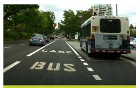
This curbside bus lane on Marine Drive in Vancouver, BC includes a priority signal and queue jump that allows buses to bypass traffic queued to cross the Lions Gate Bridge; buses carry about a quarter of peak-hour traffic on the bridge. Image from Flickr user TranBC
