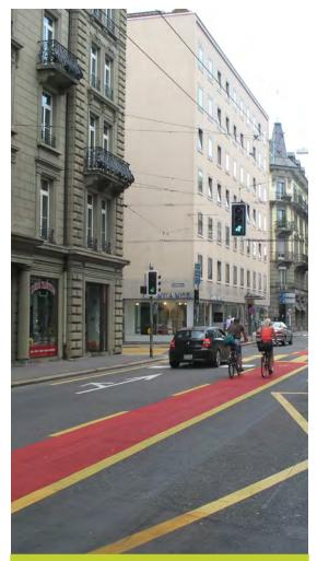
A painted bicycle lane separates this bus lane in Lucerne, Switzerland from general-purpose traffic. Yellow pavement markings within the bus lane provide further delineation.
