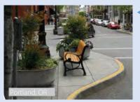
Curb Extensions: Curb Extensions: On streets with on-street parking, underutilized pavement at the intersection can be rededicated to expand the pedestrian realm and reduce crossing distance. Curb extensions also improve pedestrian and motorist sightlines at intersections and help manage vehicle turn speeds.
