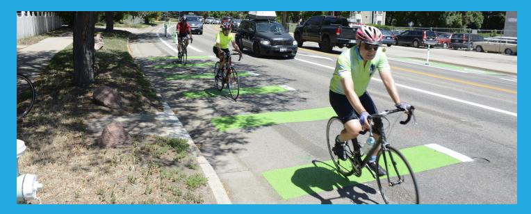
Green pavement markings: Green bike lanes were installed on Folsom Street on the northbound approaches at Canyon Boulevard and Pearl Street in September 2012. After the installation, the number of northbound right-hook collisions decreased at both locations. These markings were recently reconfigured as part of the Folsom Street Living Laboratory project. The effectiveness of green markings installed in other locations will continue to be evaluated.
