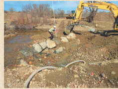
Installing j-hook
