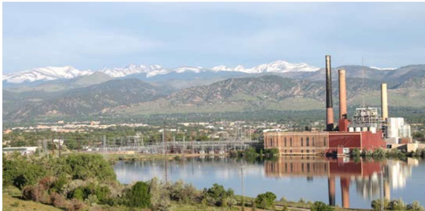
The Valmont Power Station as seen from Legion Park
