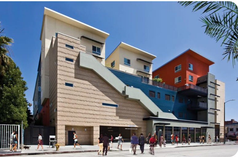
Multifamily Residential with Ground floor Retail
