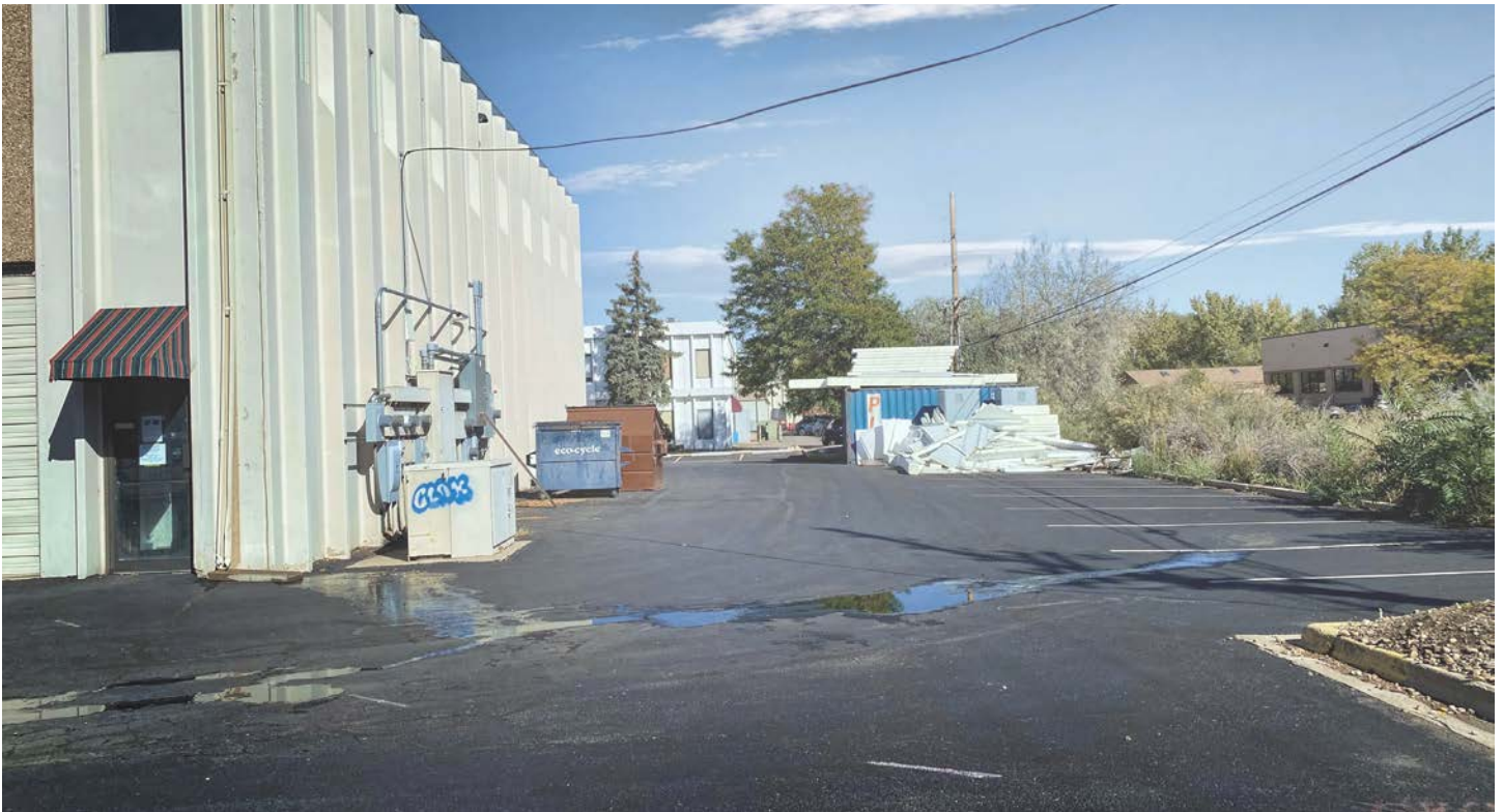
Eastern Boundary of the Station Area, Looking North – Existing Condition
