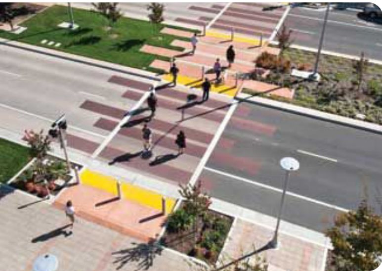
Enhanced midblock pedestrian crossing
