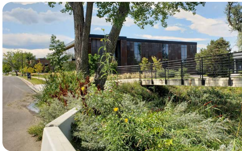
Flatirons Park Stormwater Drainage
