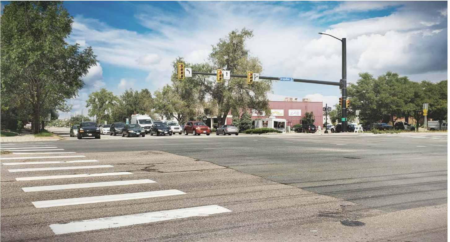
55th and Arapahoe, Looking Northeast – Existing Condition
