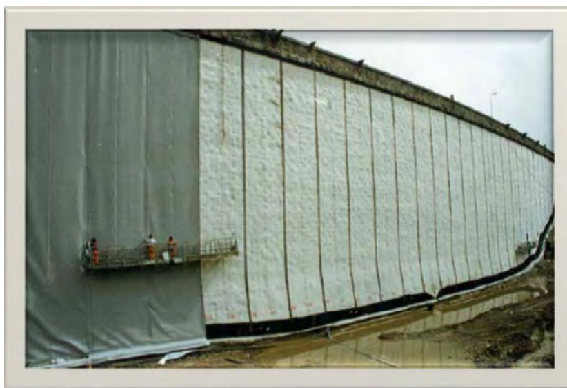
FIGURE 7-1. INSTALLATION OF GEOTEXTILE AND MEMBRANE OVER MASONRY FACE DAM 11
