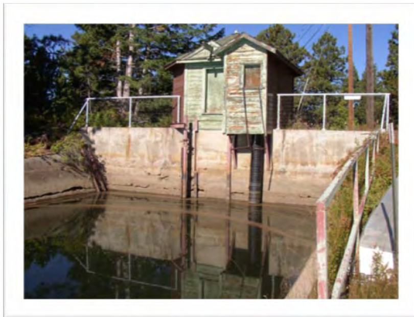
FIGURE 6-24. KOSSLER RESERVOIR GATE HOUSE AND OUTLET FOREBAY 88
