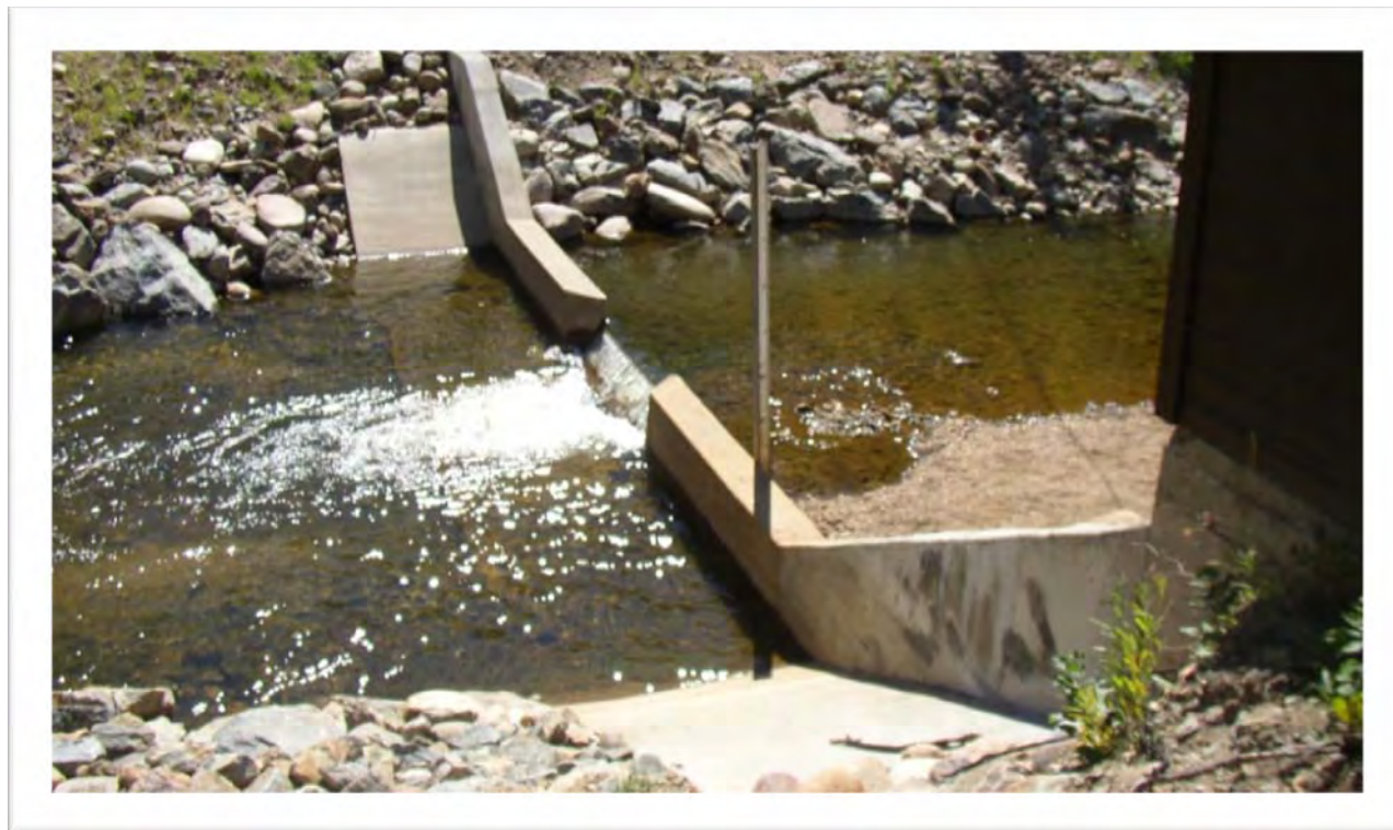
FIGURE 6-21. FLUME DOWNSTREAM OF BARKER DAM 81
