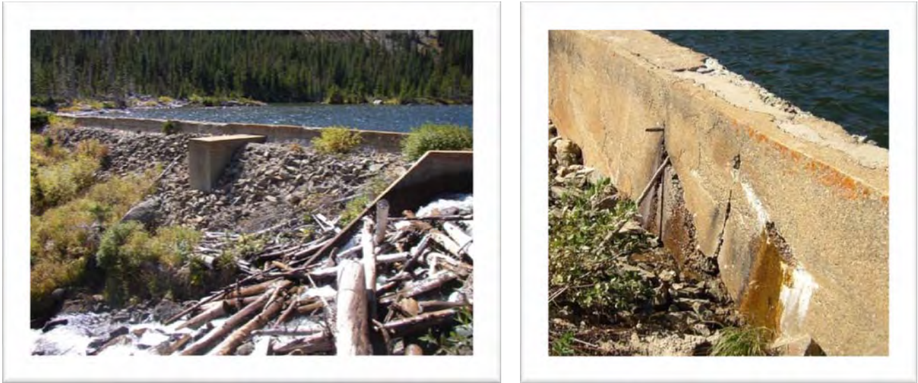
FIGURE 6-17. ISLAND DAM DEBRIS BUILDUP AND LEAK 62
