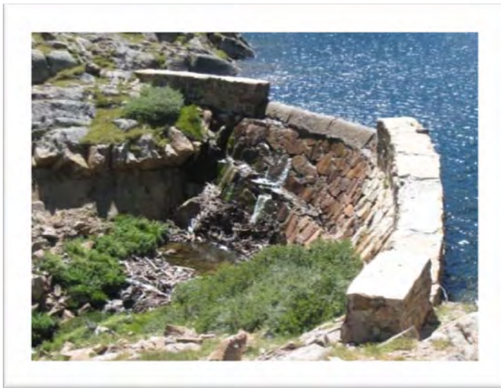
FIGURE 6-18. SEEPAGE THROUGH SKYSCRAPER DAM AND BENT OUTLET GATE STEM 74
