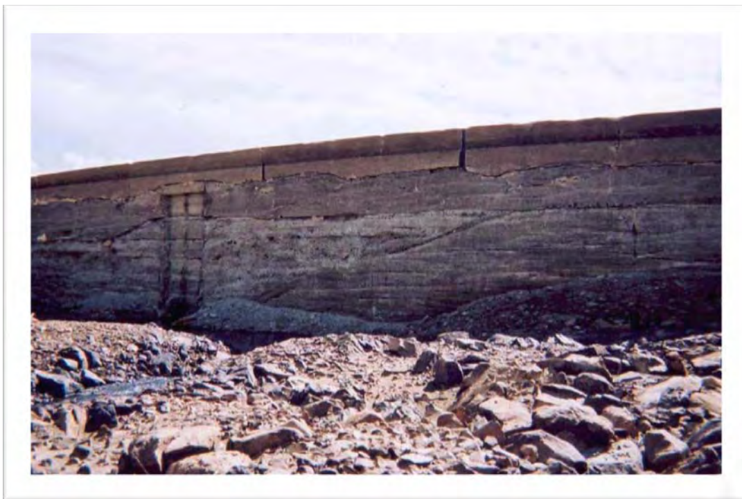
FIGURE 6-14. SPALLING AND CRACKING ALONG UPSTREAM FACE OF ALBION DAM 58
