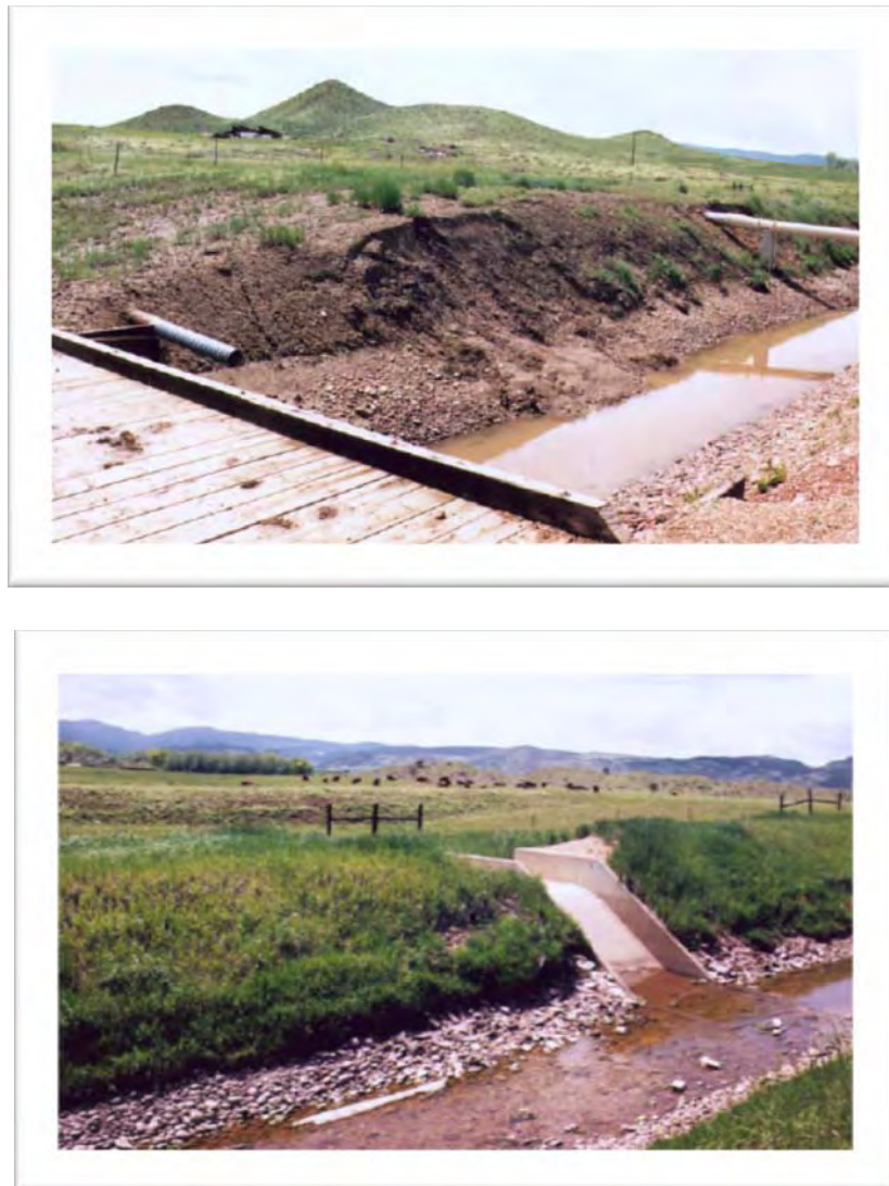
FIGURE 5-41. OUTFALLS TO BOULDER FEEDER CANAL 188
