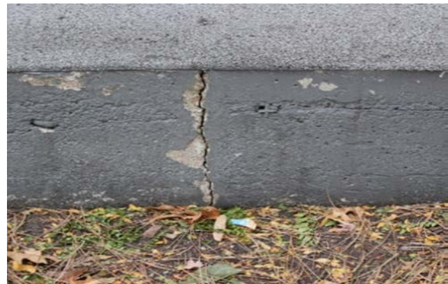
Figure 1-17. Vertical foundation crack on the east side, 2020 (source: Ratio and JVA)
