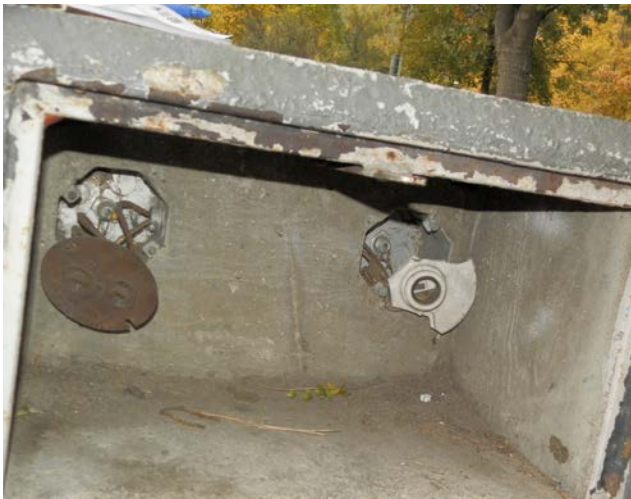
Figure 1-26. Interior view of lighting and power bollards. Note the cracking concrete forms, rusted and broken cover plates, as well as missing components, 2020 (source: Ratio)
