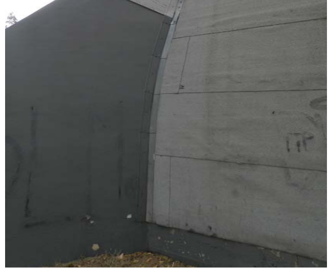
Figure 1-19. View of rolled asphalt roofing. Note the blistering at the lower portion of the roof, 2020 (source: Ratio)
