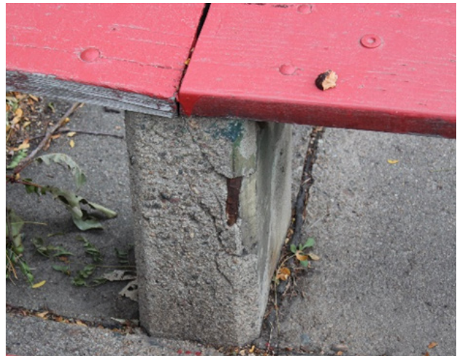
Figure 1-27. Seating showing spall at pedestal, 2020 (source: Ratio)
