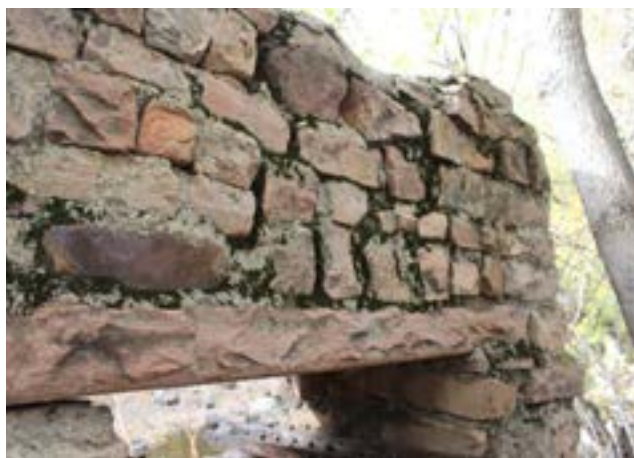
Figure 1-12. Biogrowth and areas of missing mortar, 2020 (source: JVA)
