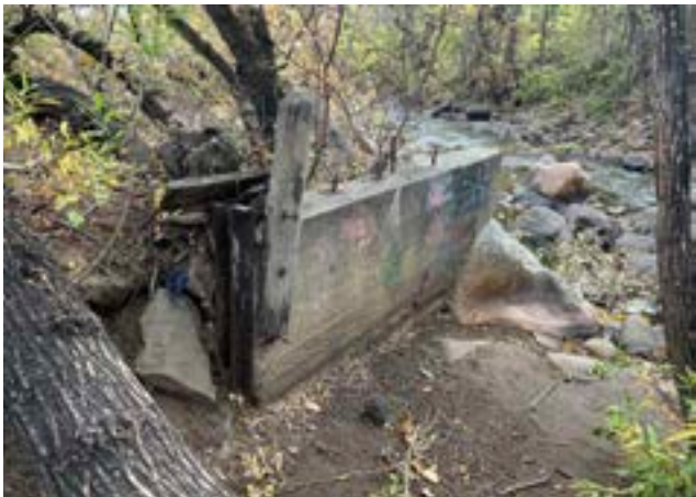
Figure 1-9. Concrete dam and headgate (source: Mundus Bishop)
