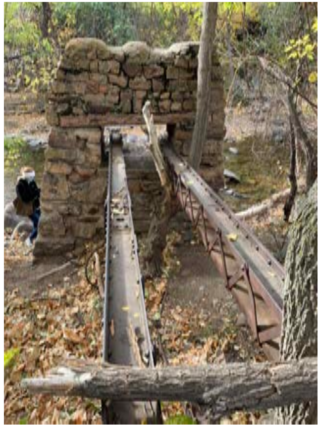
Figure 1-8. North pylon and iron support girder, 2020 (source: Mundus Bishop)
