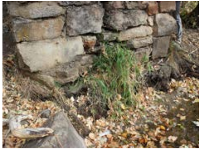
Figure 1-15. Base of north pylon. Note the scour at the creek bank's edge, 2020 (source: JVA)
