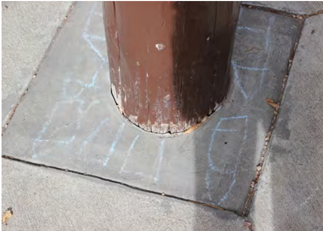
Figure 1-19. Decay at base of timber post, 2020 (source: JVA)
