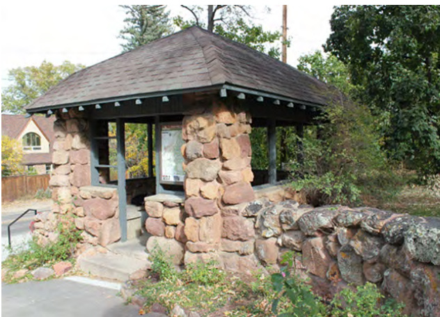
Figure 1-23. West wall showing attached retaining wall, 2020 (source: JVA)
