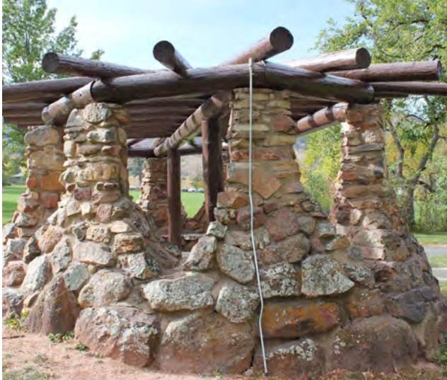
Figure 1-17. The Arbor looking West, note lichen growth and eroded mortar joints, 2020 (source: JVA)
