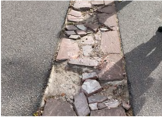
Figure 1-38. Broken stone gutter along main drive, 2020 (source: Mundus Bishop)
