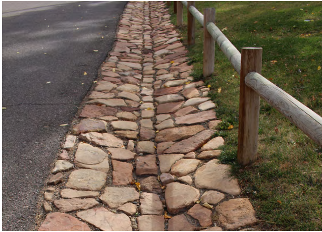
Figure 1-40. Recently installed stone gutters with compatible materials (source: Mundus Bishop)
