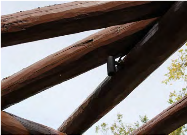
Figure 1-21. Interior lights hidden in timbers, 2020 (source: JVA)
