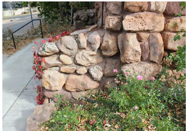
Figure 1-26. Differential settlement crack at northwest buttress, 2020 (source: JVA)
