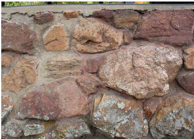
Figure 1-25. Repair mortar – note red color and separation cracks, 2020 (source: JVA)
