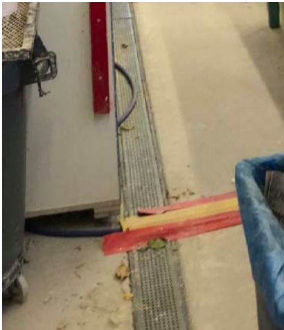
Figure 1-4. View of linear floor drain, 2020 (source: Ratio)
