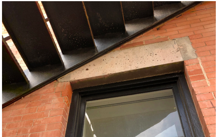
Figure 1-10. View of lintel below exterior stair, 2020 (source: Ratio)
