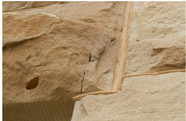
Figure 1-10. View of cracked header, 2020 (source: Ratio)
