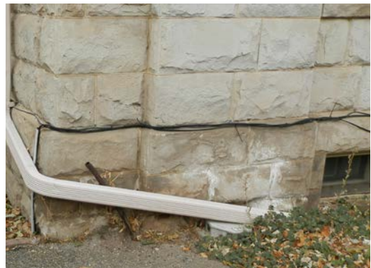
Figure 1-12. View of stone damage at gutter, 2020 (source: Ratio)
