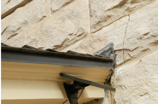
Figure 1-13. View of cracked stone, 2020 (source: Ratio)
