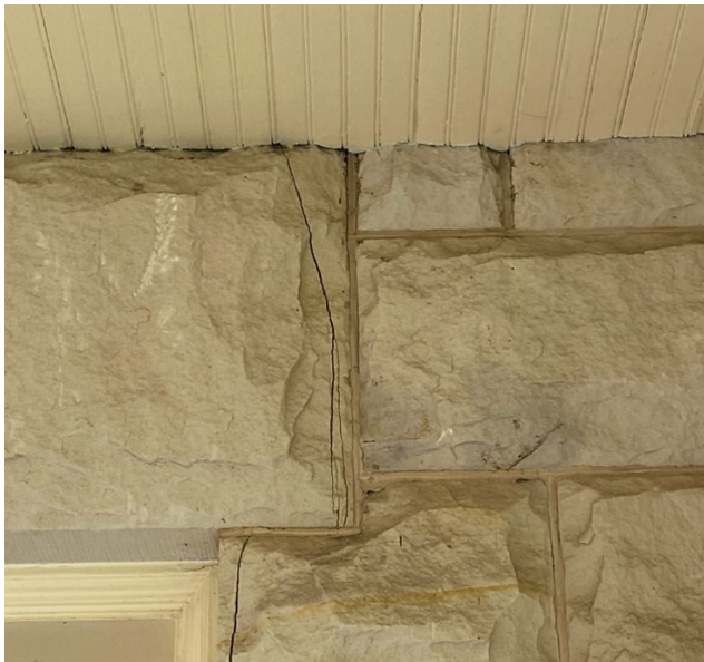
Figure 1-63. Thermal related cracking at door jamb, 2020 (source: JVA)
