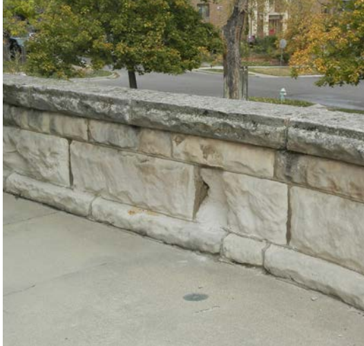
Figure 1-5. View of the stone damage at the interior porch wall, 2020 (source: Ratio)
