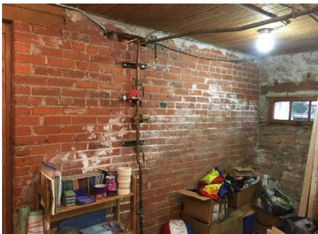
Figure 1-59. Efflorescence on basement walls, 2020 (source: JVA)
