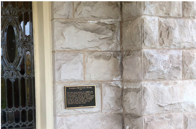
Figure 1-9. View of efflorescence west of main entry, 2020 (source: Ratio)
