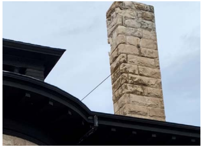
Figure 1-62. Deteriorated and loose stone at chimney
