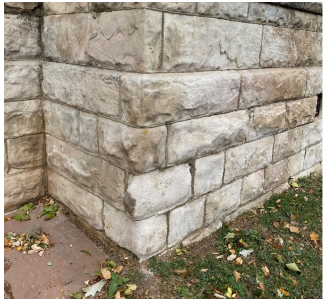
Figure 1-64. Erosion of stone near grade and lichen growth at coping, 2020 (source: JVA)
