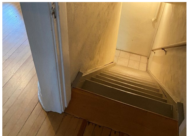
Figure 1-60. Horizontal bulge in basement stair wall, 2020 (source: JVA)
