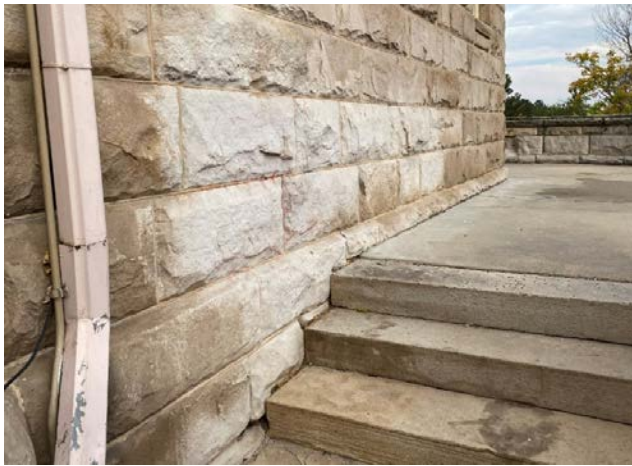
Figure 1-61. Erosion of stone at locations of graffiti removal, 2020 (source: JVA)
