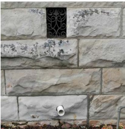
Figure 1-16. View of lichen and weathered stone, 2020 (source: Ratio)
