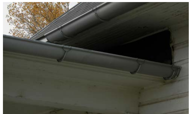
Figure 1-18. View of half-round gutters, 2020 (source: Ratio)
