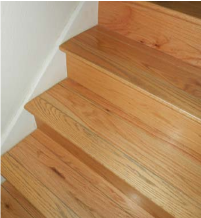
Figure 1-14. View of wood treads and nosings, 2020 (source: Ratio)
