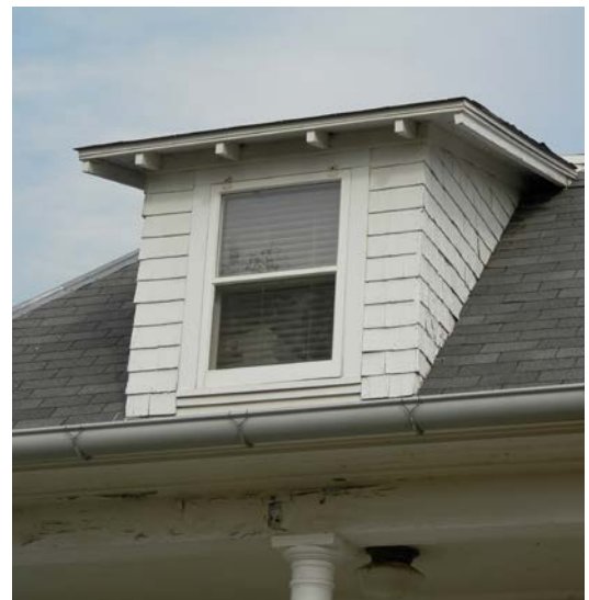
Figure 1-16. View of the wood shingled dormers, 2020 (source: Ratio)
