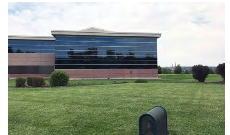
Suburban-style office park in East Boulder with significant turf area
