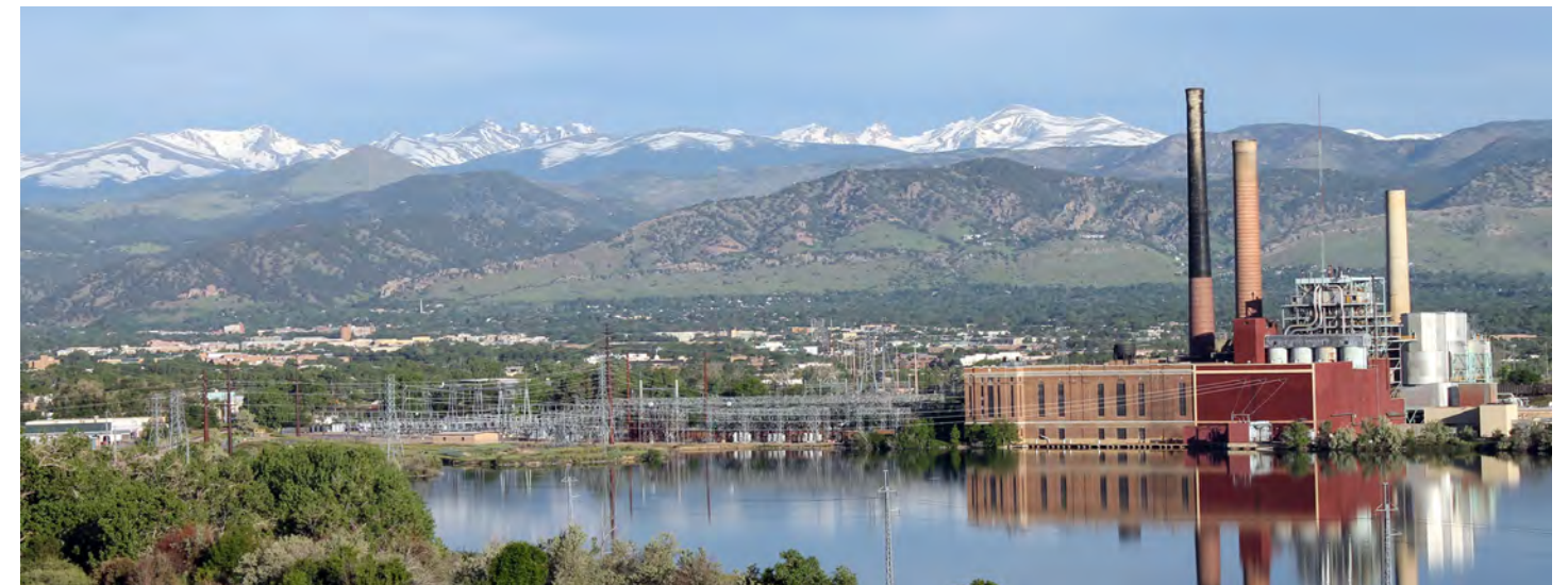
Valmont Power Plant
