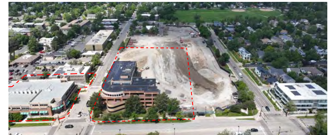
EXISTING CONDITIONS - HOSPITAL DEMOLITION COMPLETED
