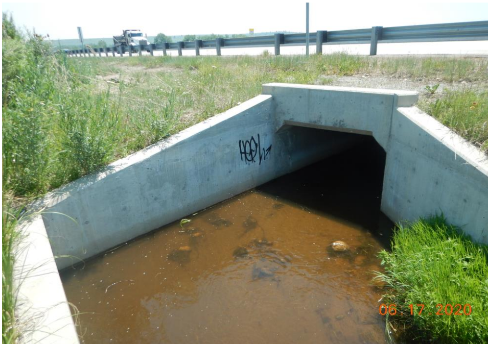
Photograph 2: DCD2 box culvert on north side of US36 discharging to concrete-lined channel, looking south.
