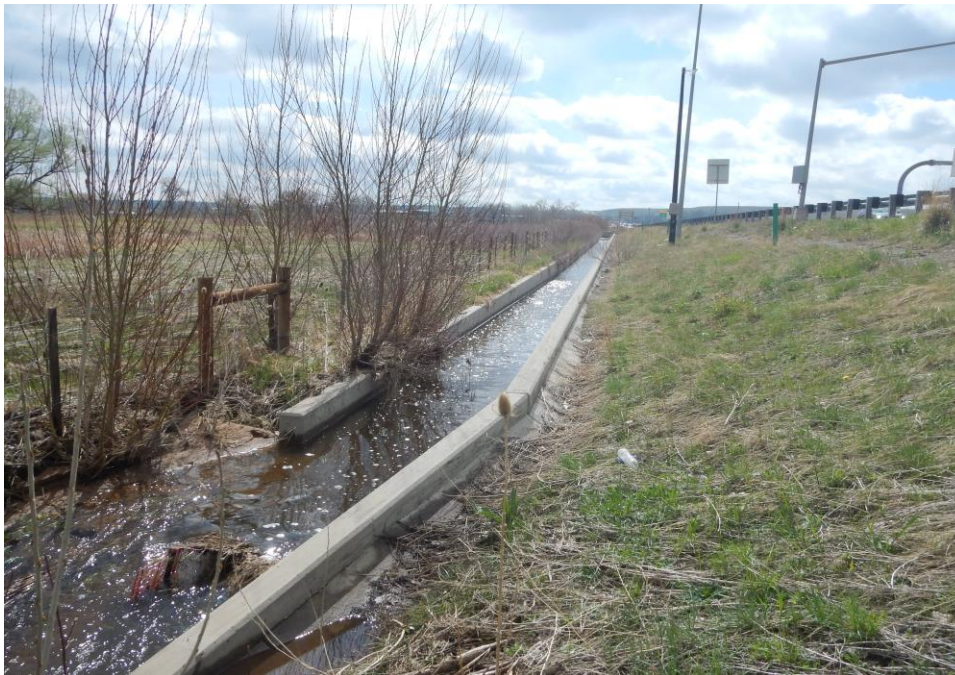
Photograph 4: DCD2 concrete lined channel transitioning to earth ditch north of US36, looking east.
