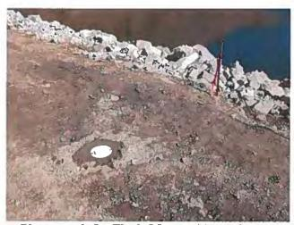
Photograph 5 - Flush-Mounted Well Casing
