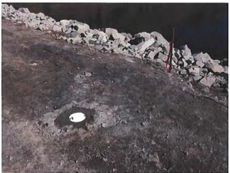
Photograph 2: Flush-Mounted Well Casing.
