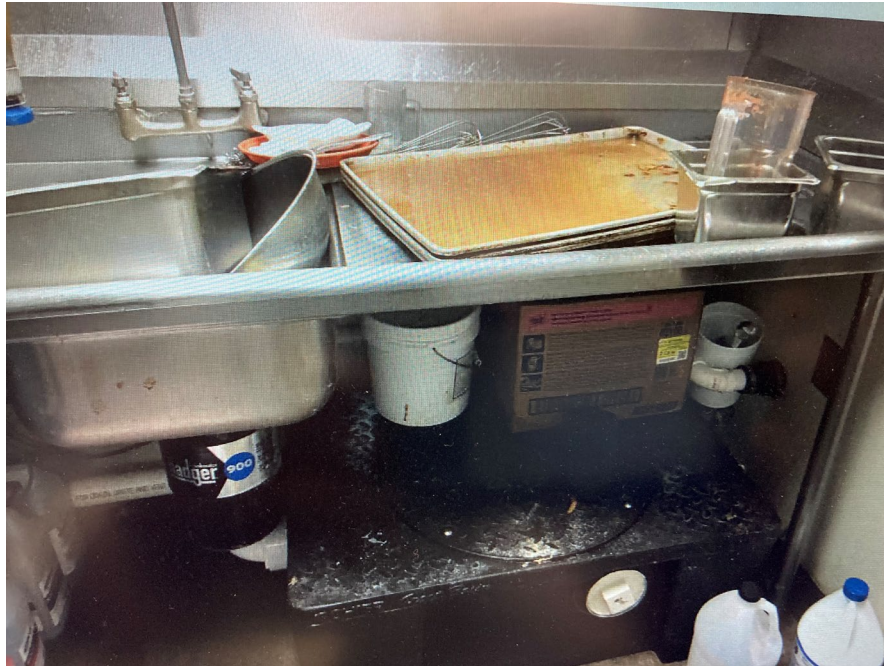
HGI retrofit under dishwash sink.
