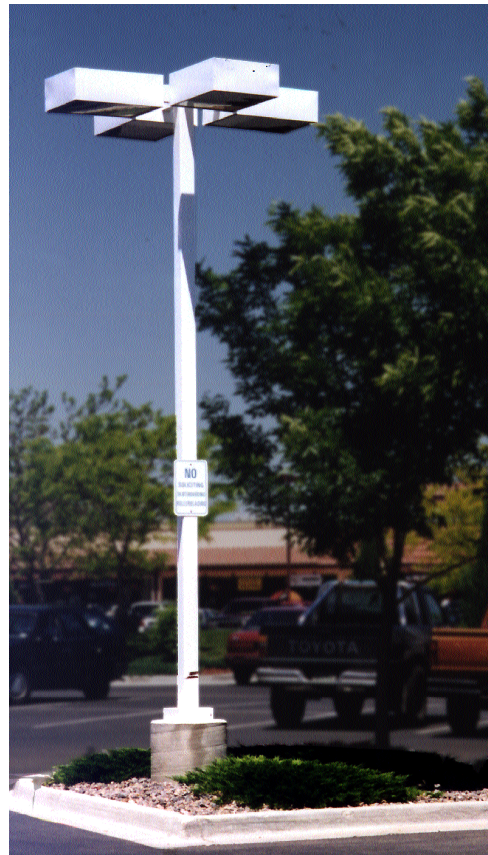
▲ 3.5.L. Parking lot fixtures should be proportionate to the height of the building and size of the parking lot.
