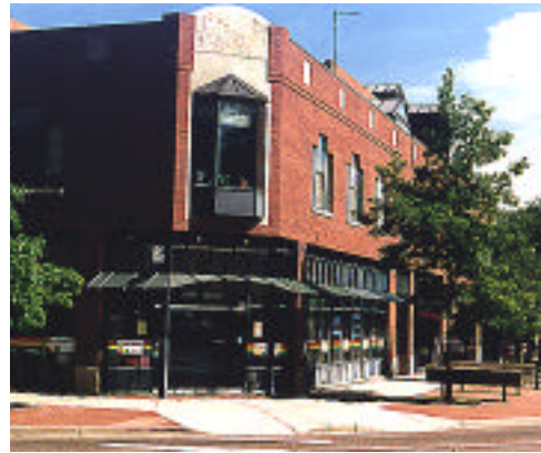
▲ 3.5.F. This parking garage is wrapped by retail on the first floor and offices on the second.
