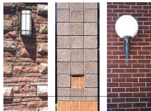
▲ 5.2.I Stone, brick and small concrete blocks are modular building materials that have a human scale.
