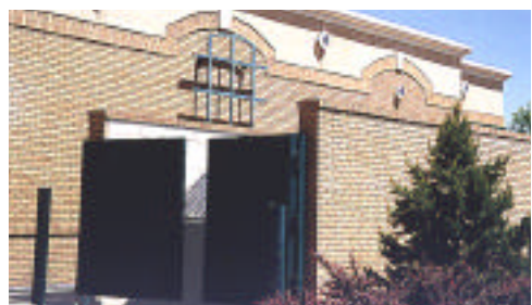
▲ 5.3.C. This trash storage area is enclosed by a brick wall that matches the building facade.
