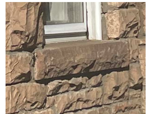
Stone Lintels and Sills
