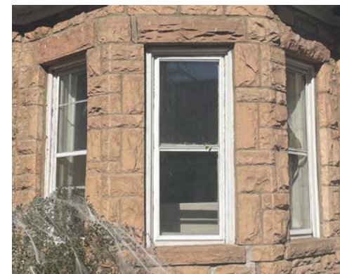
White Painted Windows and Doors
