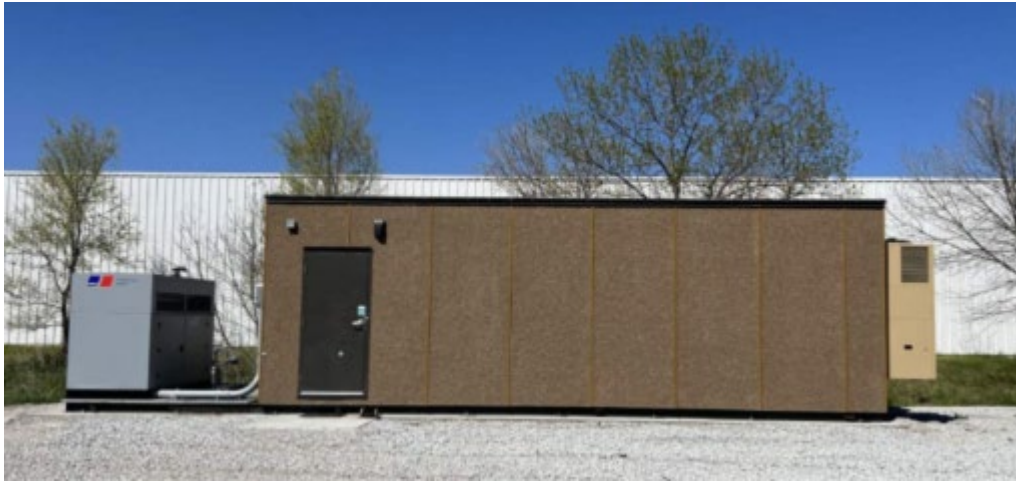
Figure 5. Sample Image of Structure
