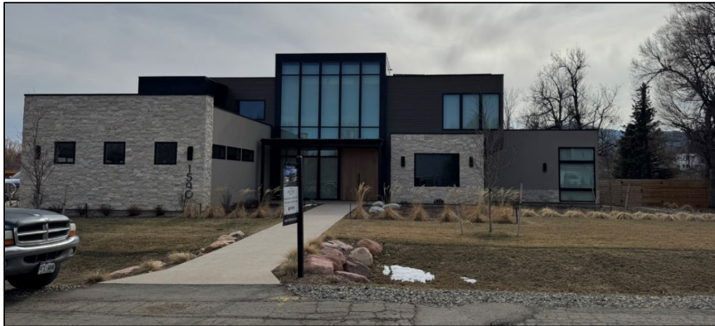
Figure 1: Recently Completed Replacement Home
