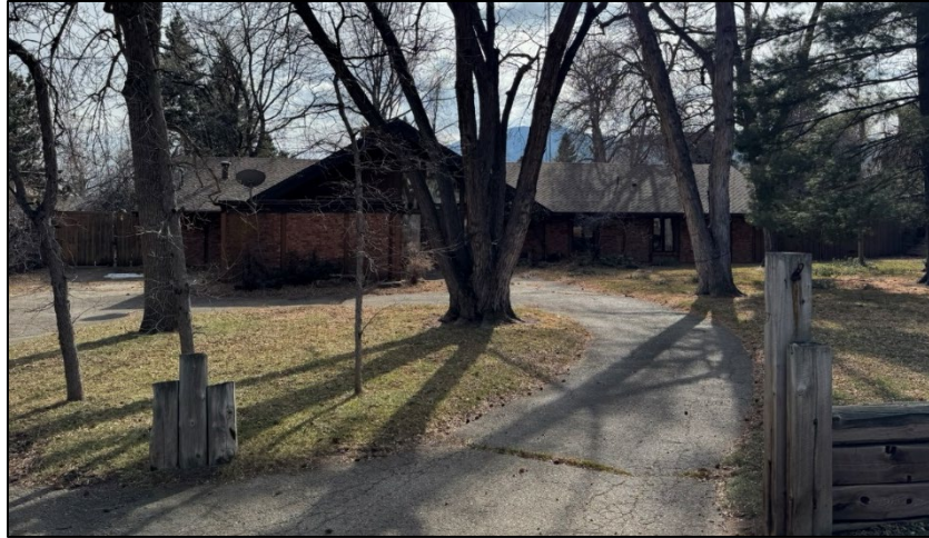
Figure 3: Home Approved for Demolition and Replacement
