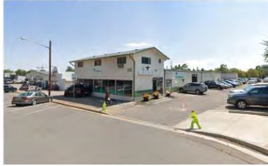
Previously Hoshi Motors
