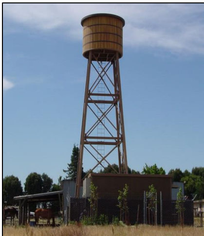
Example of creative stealth screening of antennas.
