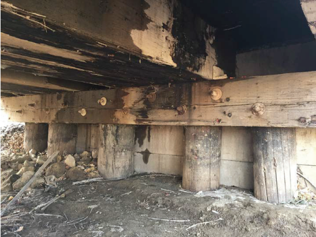
Typical Abutment Bent
