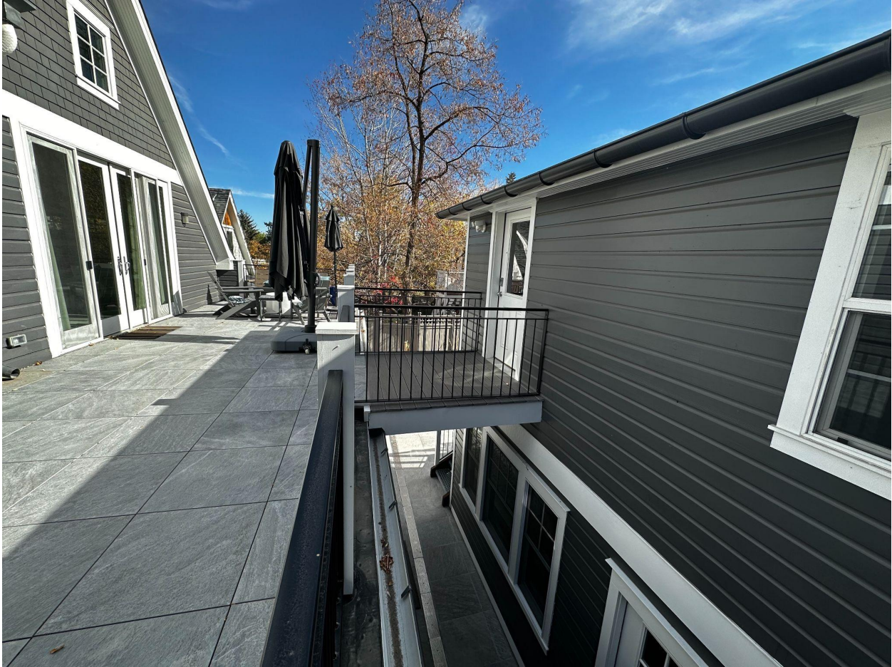
Existing Bridge Connection Facing East
