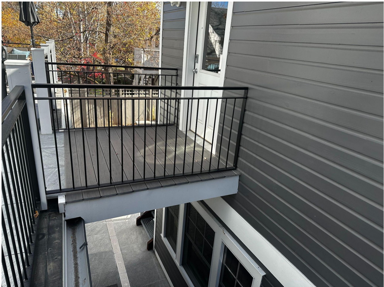
Existing Bridge connection between patio deck and garage (facing East)
