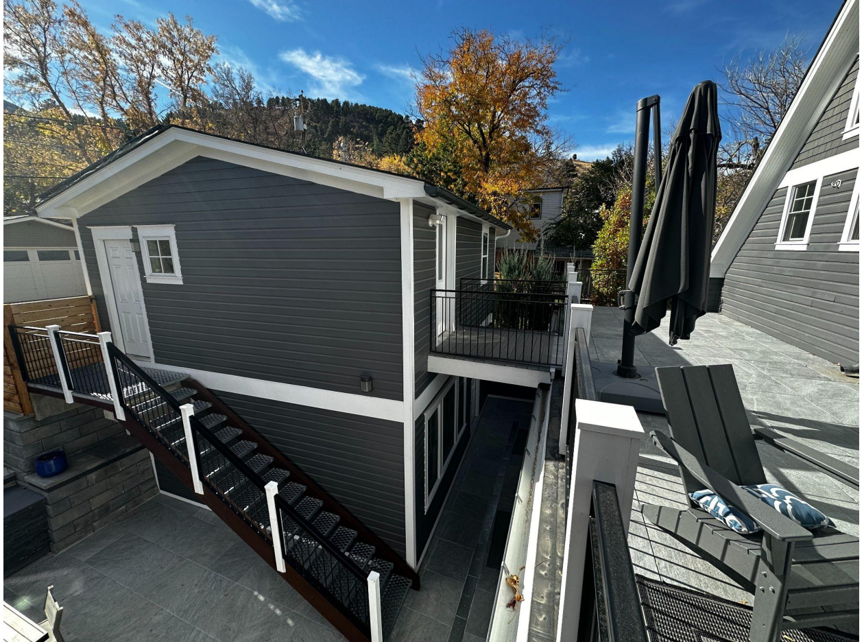
Existing Bridge Connection Facing West
