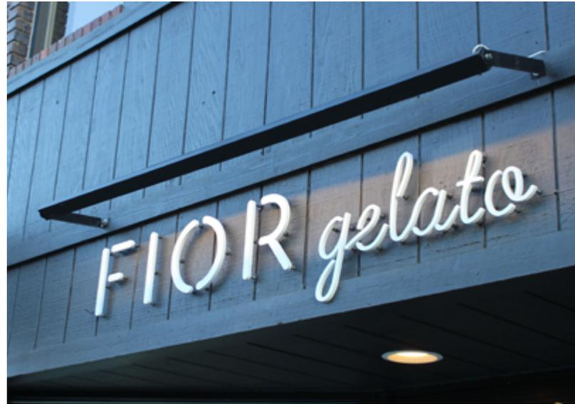
Fig. 18 Wall sign with shielded external luminaire
