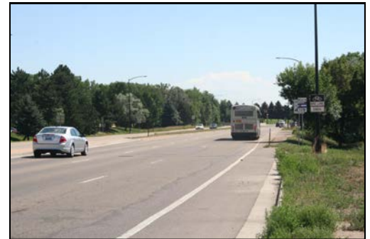
Existing conditions at Diagonal Highway between 28 th & 30 th Streets.
