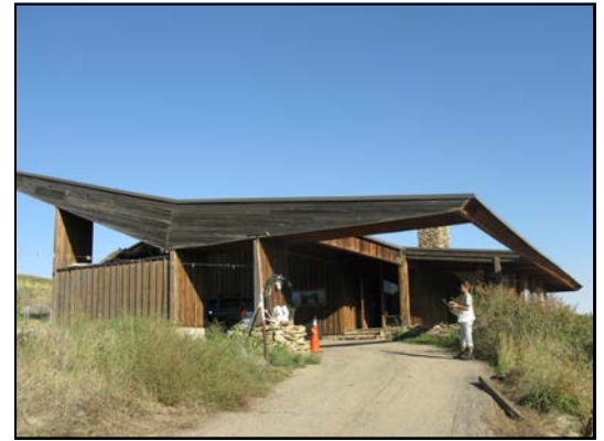
Viele House prior to repairs
