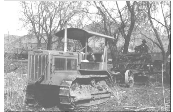
Construction of Central Park, 1929. Photo Courtesy the Carnegie Branch Library for Local History
