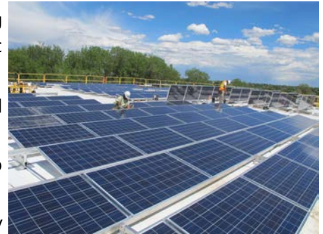
Solar panels at the OSMP Ute Annex office building
