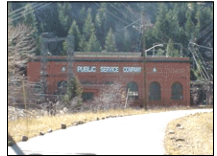
Boulder Canyon Hydroelectric Facility
