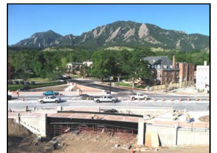
Construction of the Broadway underpass at Euclid Avenue
