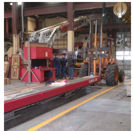
New vehicle lift at Fleet Services
