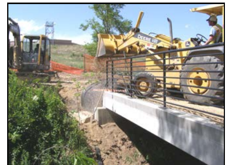
Construction of a bridge at Valmont City Park
