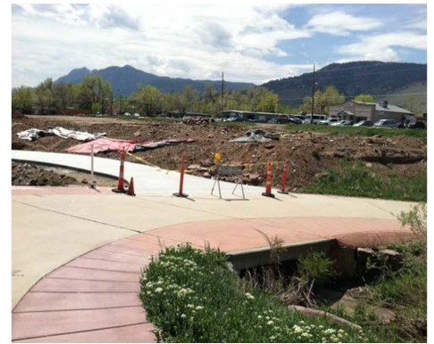
New multi-use path constructed in conjunction with the Violet Crossing development
