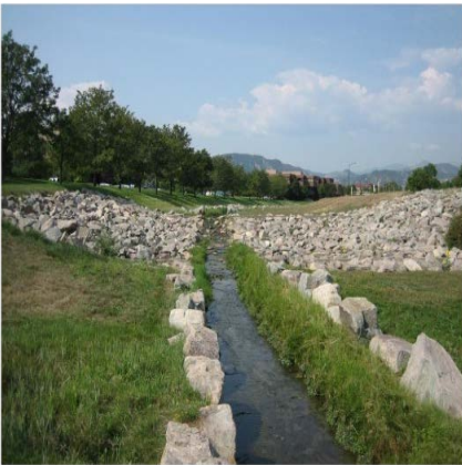
Goose Creek restoration project will begin in 2012.
