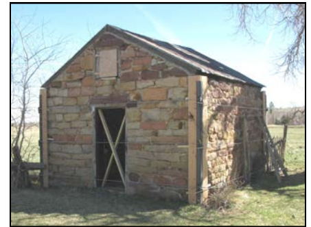
Hedgecock Shed Repairs
