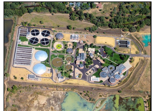
75th Street Wastewater Treatment Plant
