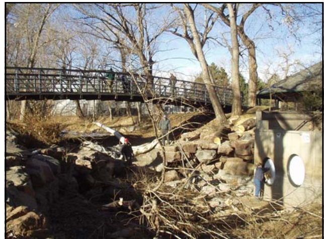
Work on Boulder Creek at the Fish Observatory.
