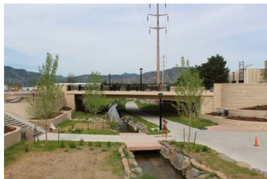
Boulder Junction Improvements at Junction Place and Goose Creek.
