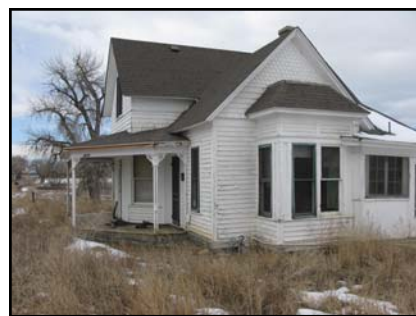
Hartnagle Homestead after restoration.
