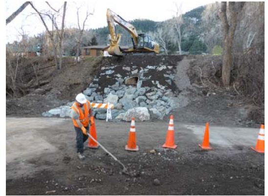
Stream bank restoration work on Boulder Creek at Eben Fine Park.
