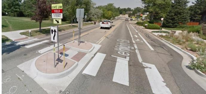
A photograph of a residential street with an enhanced pedestrian crosswalk. The crosswalk features a central median refuge with a red brick border and a white top. A white sign with a black arrow pointing up and a black silhouette of a pedestrian is posted on the median. A yellow diamond-shaped sign with a black border and a black silhouette of a pedestrian is also visible on the left side of the road. |
