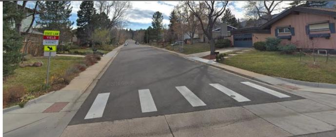
A photograph of a residential street with a standard marked crosswalk. The crosswalk consists of white parallel stripes across the road. A yellow diamond-shaped sign with a black border and a black silhouette of a pedestrian is posted on the left side of the road.                                                                                                                                              |
