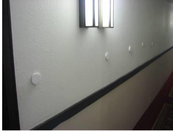
Drill & Fill Wall Insulation
