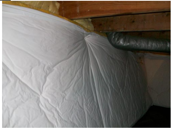
Crawlspace Foundation Wall Insulation
