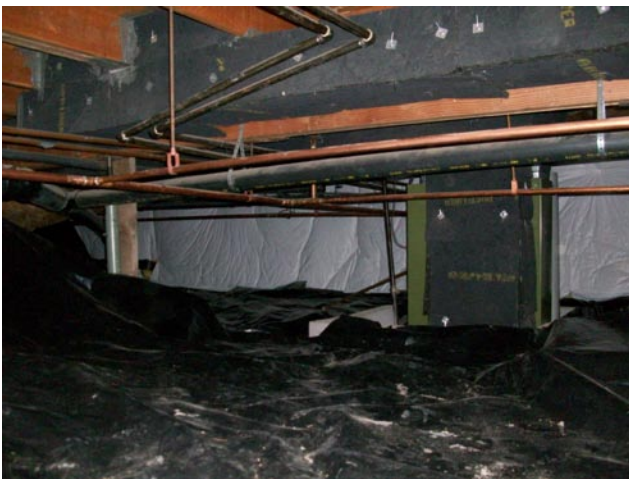
Crawlspace Vapor Barrier
