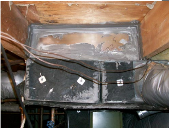
Duct Sealing
