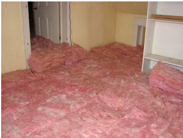
Fiberglass insulation in Attic
