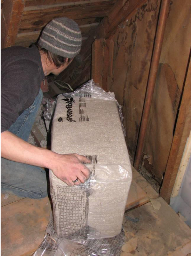
Loose Cellulose in Attic
