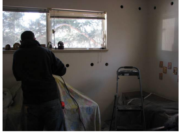
Drill & Fill Wall Insulation
