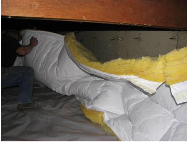
Crawl Space Wall Insulation
