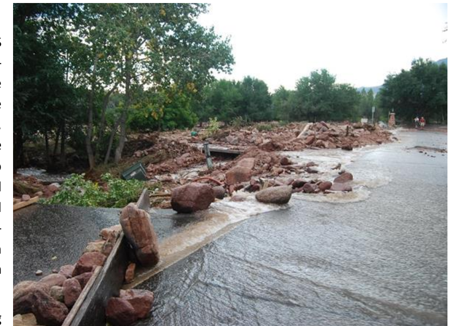
2013 flooding damage at Spring Valley Road and Linden Avenue
